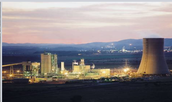
Siemens IGCC in Puertollano (E)
