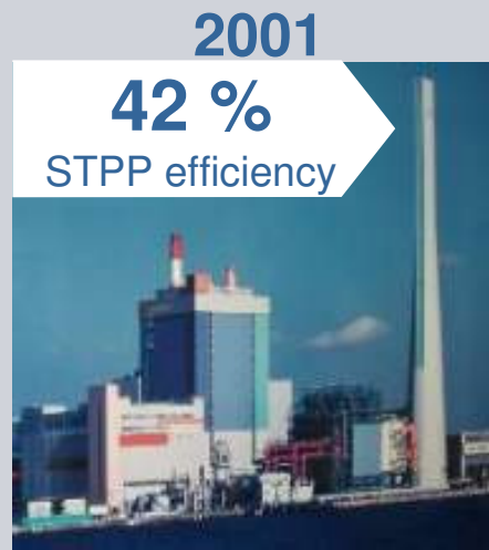
STPP Isogo 1 designed for 600 MW
