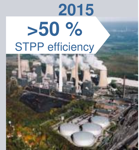
STPP 50plus (E.ON) designed for 500 MW
