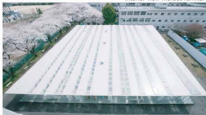
view of the roof top
