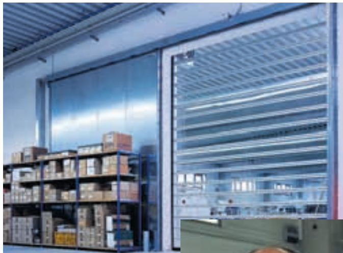
The transparent slats in the high-speed turbo-door guarantee clear visibility and reduce the danger of accidents at doors with frequent two-way traffic.
