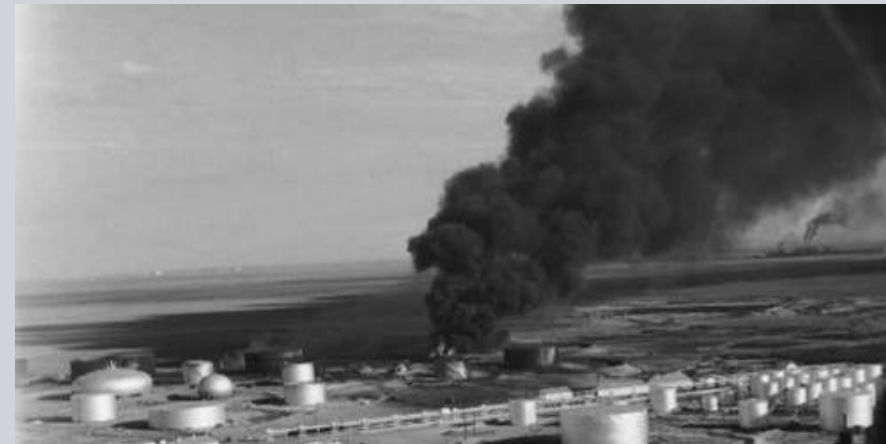
Tank farm explosion near Dumas, Texas
